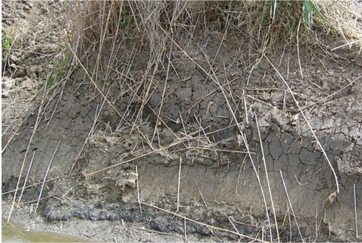
Figure 2. Phragmites roots and rhizomes exposed by excavations for the inlet channel. The channel is approximately 1 m deep.
