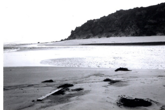
View looking across sand-bar from left bank. Note opening to sea. During the inspection the tide turned and sea water commenced to flow upstream.
