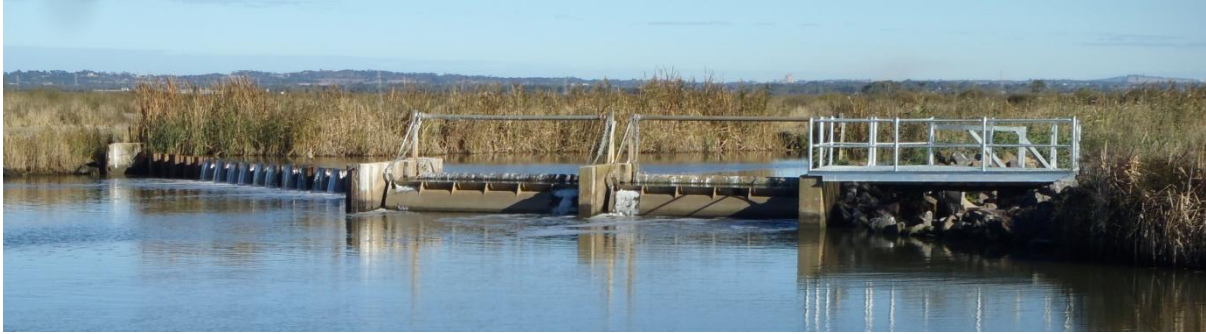
Figure 8. The Lower Barrage in the river stops sea water from moving upstream.
