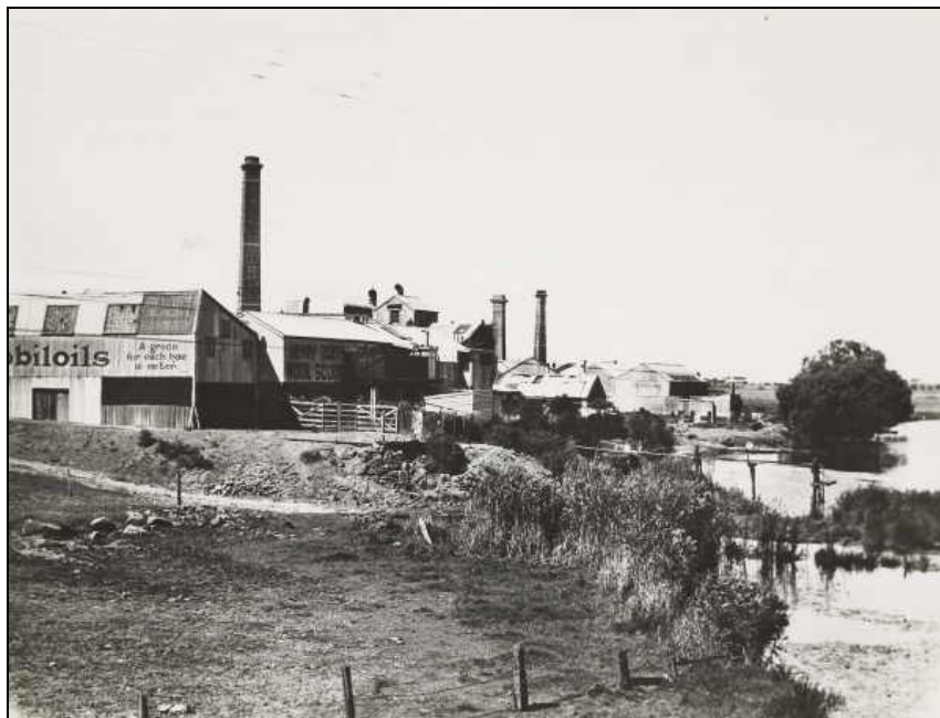
Figure 2-4. Tannery, fellmongery and O’Berne Wool Scourer, Breakwater.
