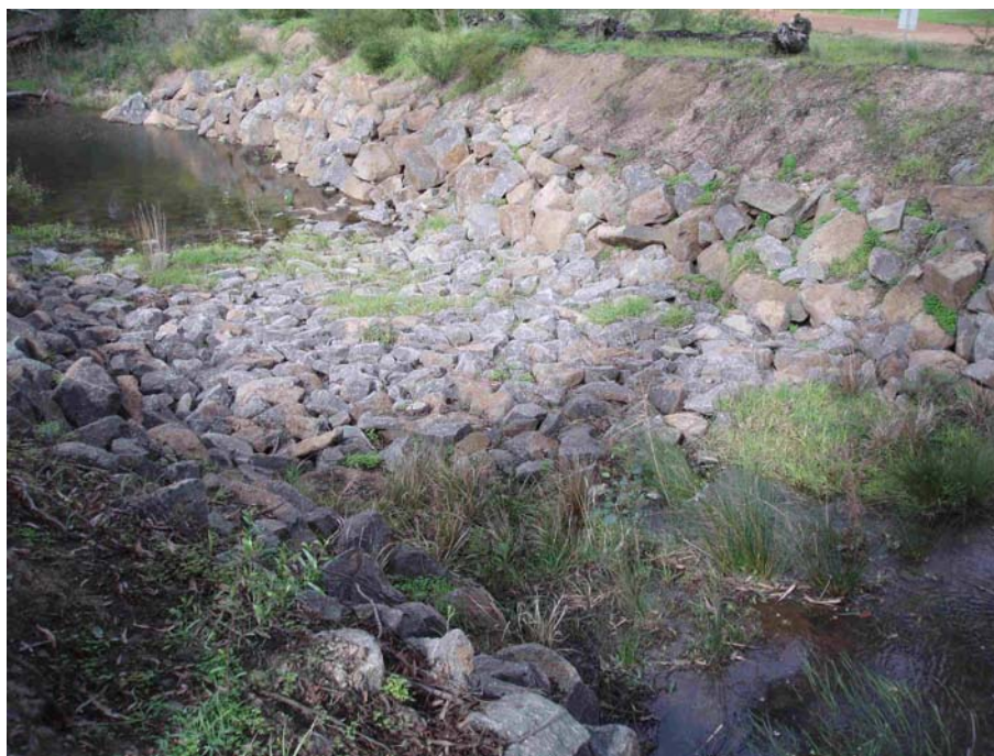
Figure 7.2. Grade control structure downstream of Old Coach Road, showing no surface water on the structure, despite flows upstream of the structure (Photo: G. Vietz).
